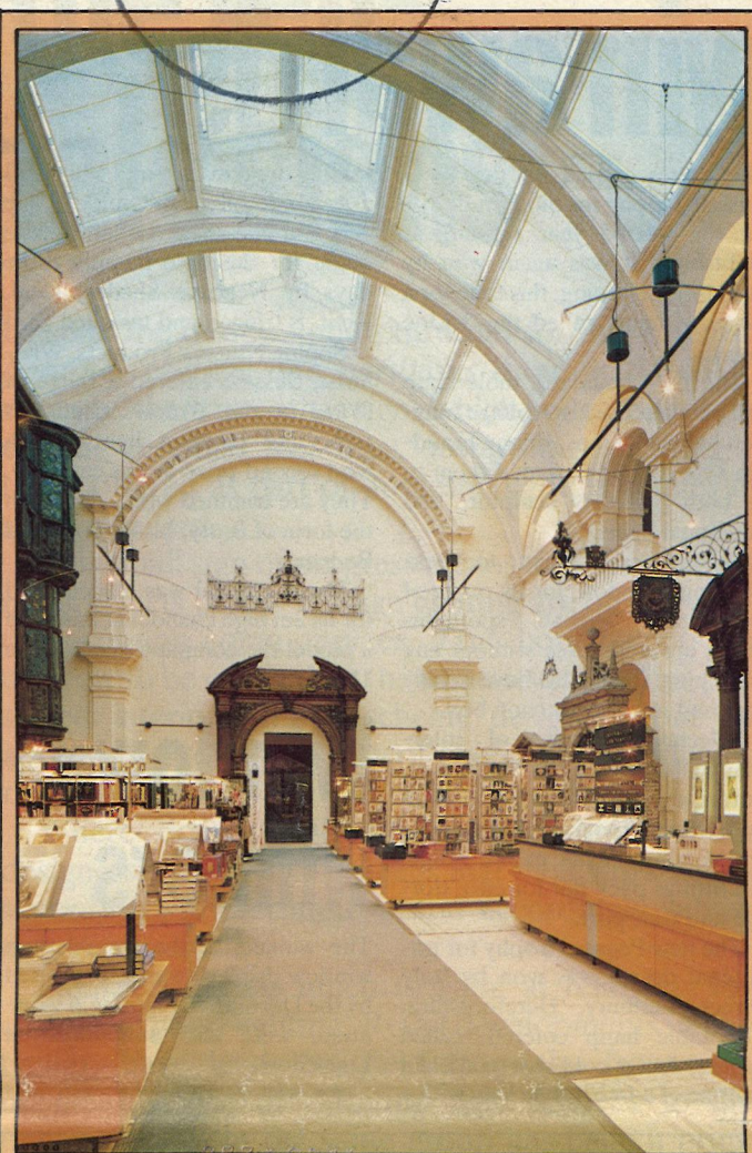
Unusual lighting has been installed in the Victoria and Albert Museum, London. It had to be unobtrusive and Microlights evolved a suspension system that is unsupported from both ceiling and floor. Six free hanging units are rigged across a 10m span on stainless steel wires. Each holds eight 75W low voltage miniature tungsten halogen lights.
