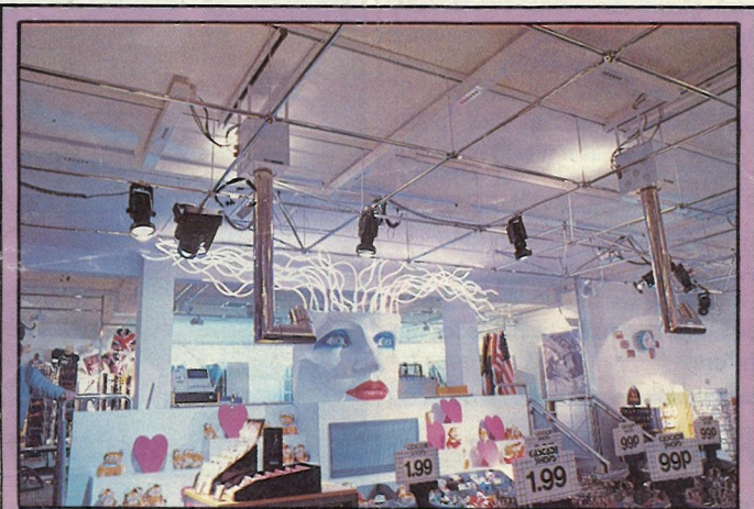
In-store, light entertainment has reached an advanced stage at Cascade's latest shop in Carnaby Street, London. The low voltage lighting scheme installed by Classic Electrical Contractors offers 90 different programmes. As well as moving disco lighting effects there is a huge face with neon tubing hair.
